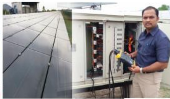
PQ Audit at 1MW Grid Integrated Solar Power Plant
