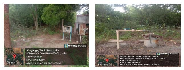
This bore well is located into an underground in the various places of our campus such as Backside of Automobile block, Nearer to Indoor Stadium, At Gents hostel, Nearer to College main gate etc . The 5HP electrical pumps are used in our campus to pump out the water from the bore wells.
